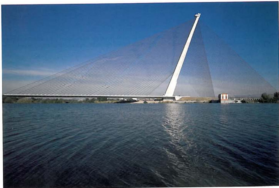
Figura 1. Alzado general del puente terminado Figure 1. Elevation view of the finished bridge
