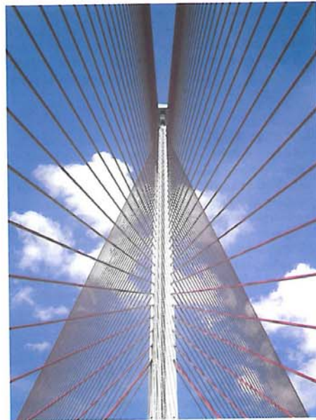
Figura 42. Alzado frontal del pylon con los 152 tirantes Figure 42. Front elevation view of the pylon with its 152 stays
